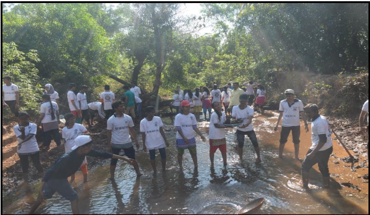
Construction of Vanrai Bandhara
