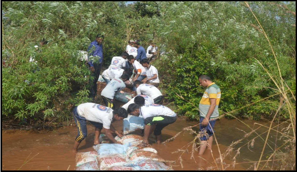
Construction of Vanrai Bandhara
