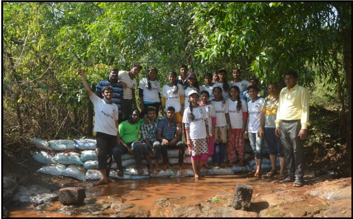
Construction of Vanrai Bandhara
