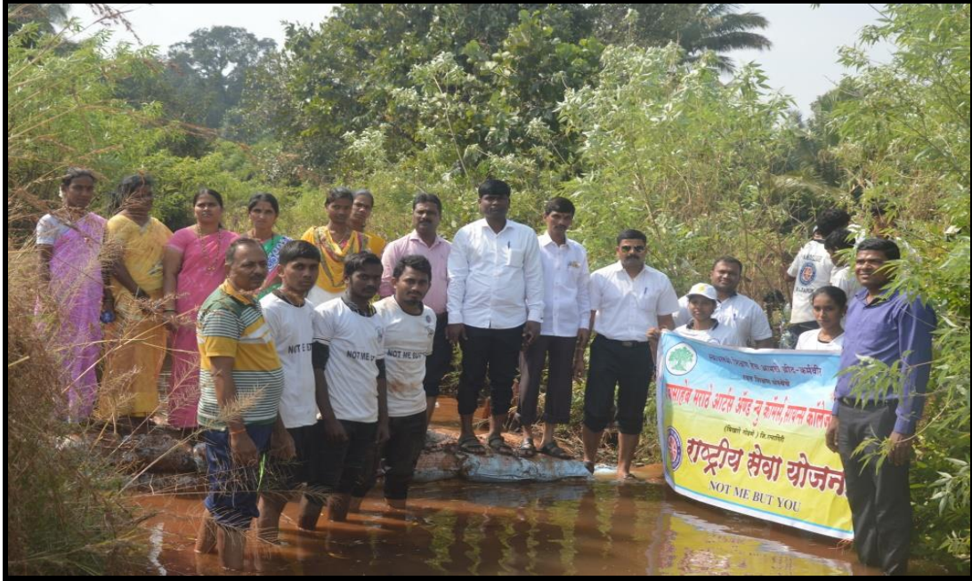
Construction of Vanrai Bandhara
